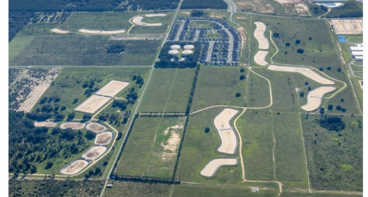
Water Conserv II infiltration Basins
