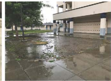
Existing site in storm event conditions
