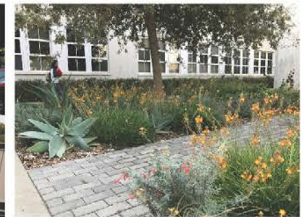
Pervious paver pathway
