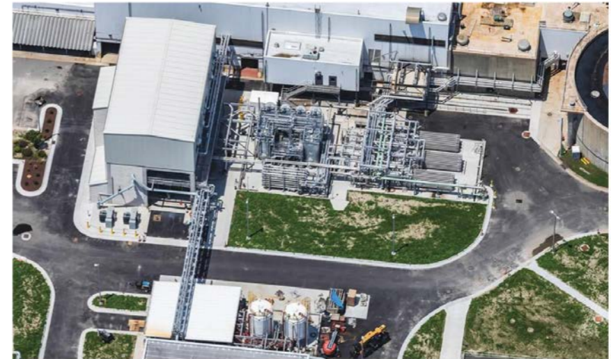
The thermal hydrolysis process (THP) system allows the Hampton Roads Sanitation District (HRSD) in Virginia to generate power and fine fertilizer directly from sewage
